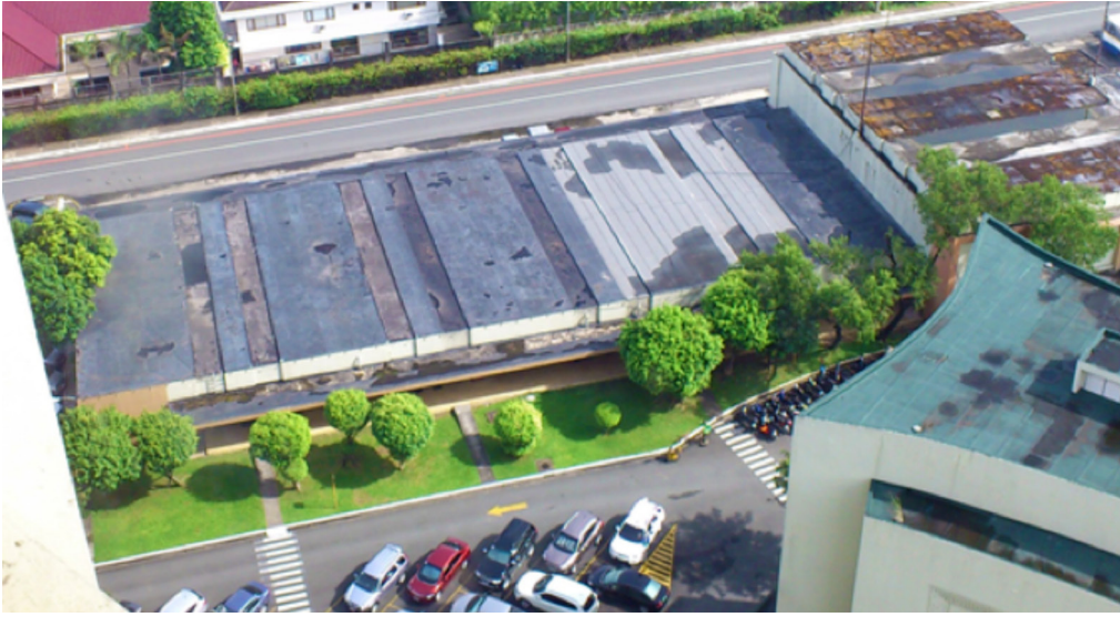
FIGURE 1.1 Aerial view of Operations Building
